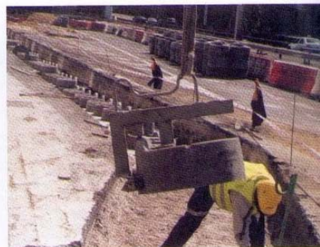
Photo 1 Manutention des cellules béton Handling the concrete cells
