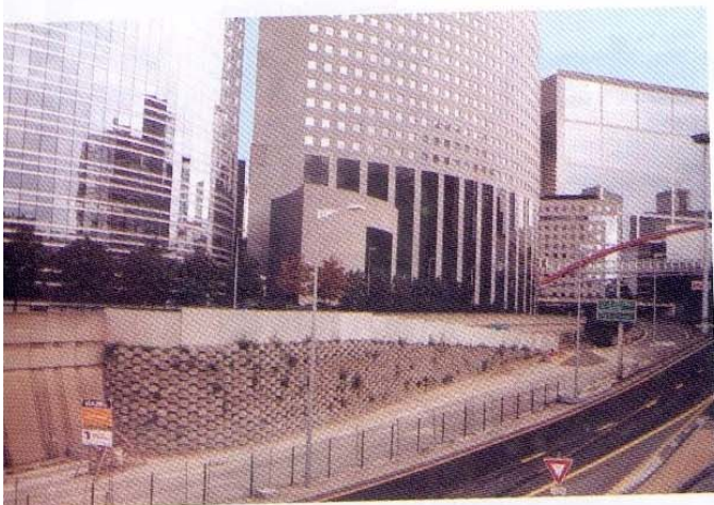
Photo 5 Vue globale de l'ouvrage fini Overall view of the finished structure
